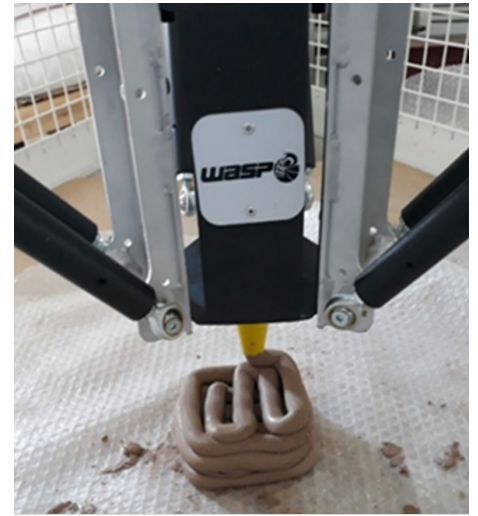
Test trials on 3D printing process with the new equipment installed at Frederick Research Center (FRC)
